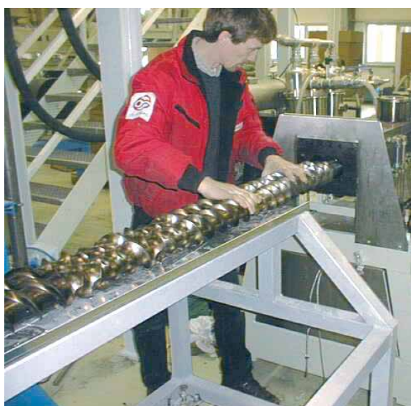
Figure 2: Installation of new extruder screws
