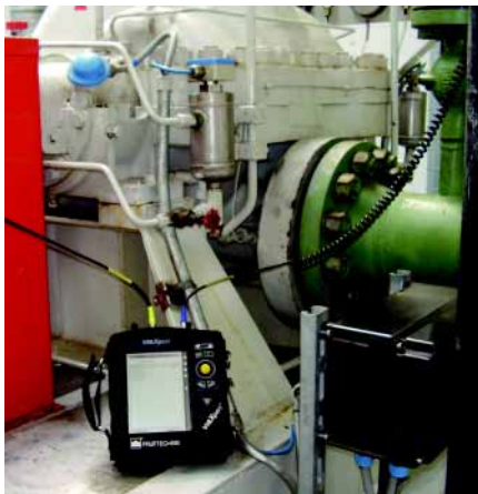
Fig. 2: Vibration measurement with VIBXPERT®
