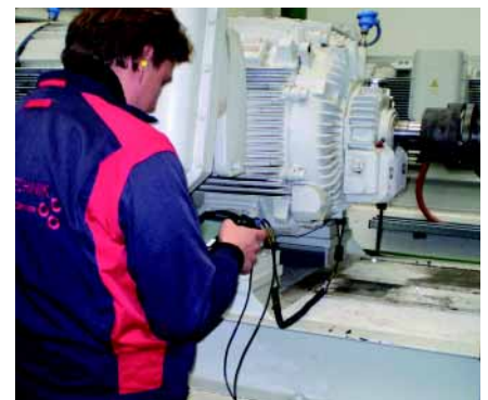
Fig. 8: Employee of PRÜFTECHNIK Machinery Service working at precision balancing the machinery
